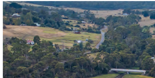
Craigburn Road continuing into Johnstons Road. Bridge and Egg Island Creek in view.
