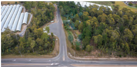
Intersection of the East Tamar Highway & Hillwood Jetty Road. Bus stop for metro services.
